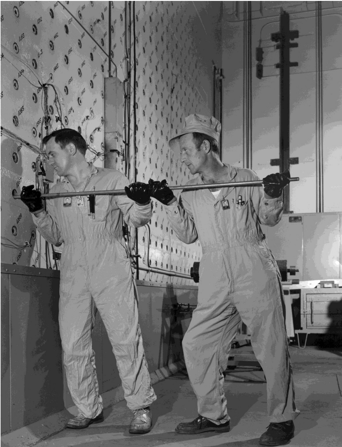
The uranium fuel being inserted into the Graphite Reactor face
